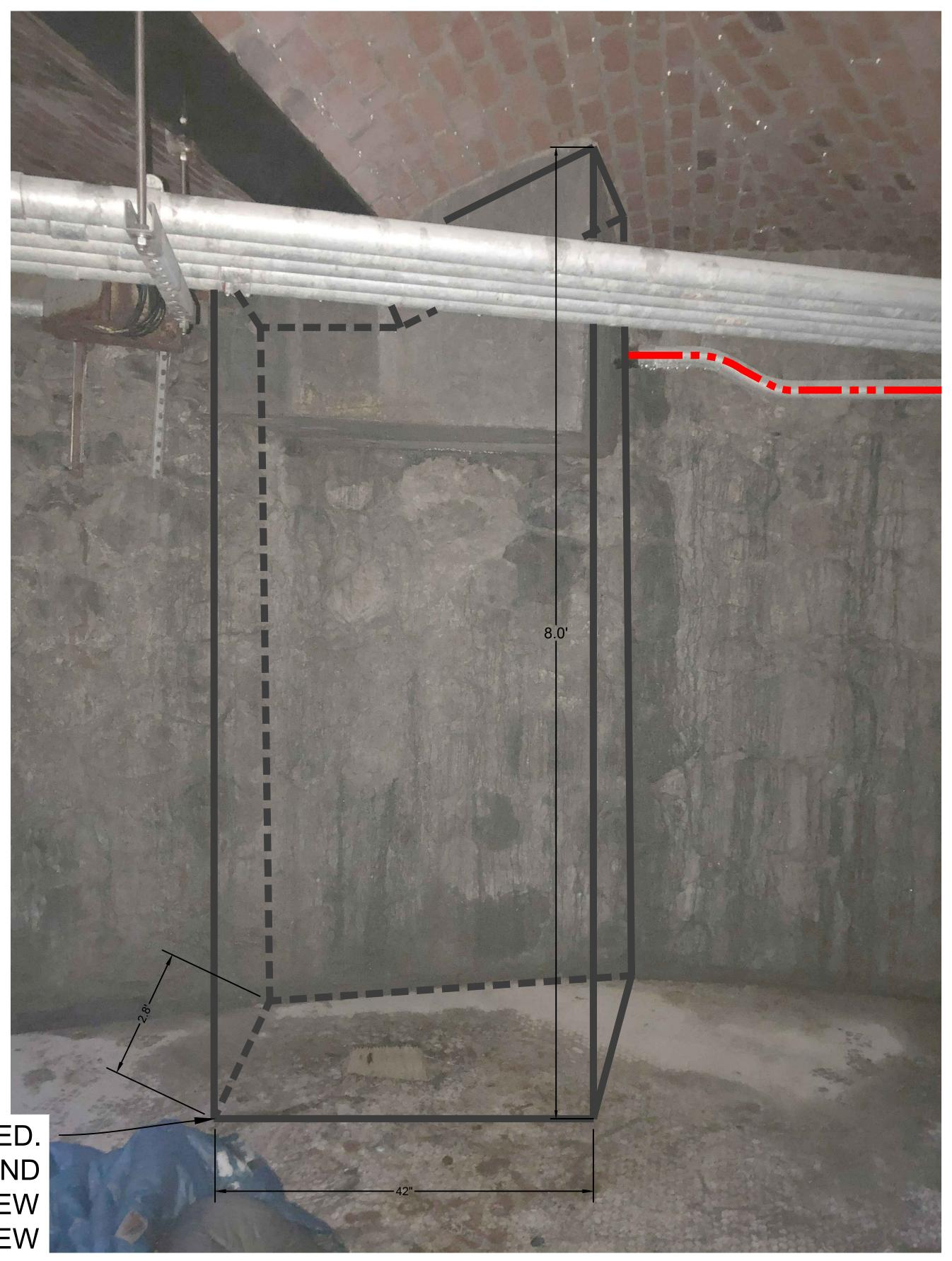
EXISTING FOUNDATION TO BE REMOVED. CONCRETE FORMS TO BE BUILT AND REMOVED AFTER CONSTRUCTION. NEW FOUNDATION TO BE SET IN NEW CONCRETE PILLAR TO THE FLOOR.
